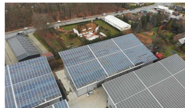
Solar panels that power the facility
