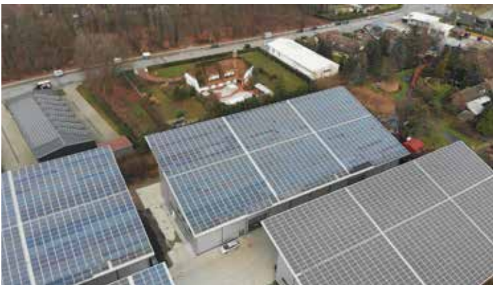
Solar panels that power the facility
