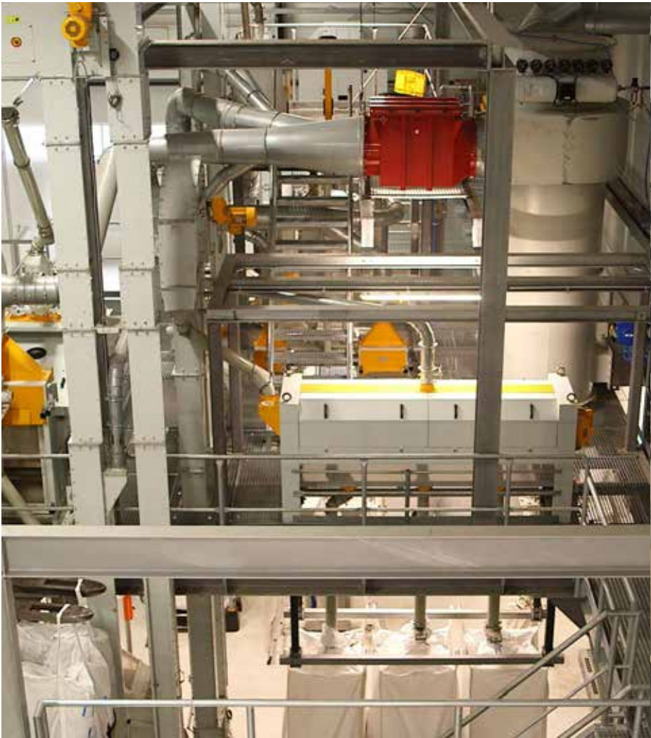
The facility is the biggest hemp food processor in Central Europe.
