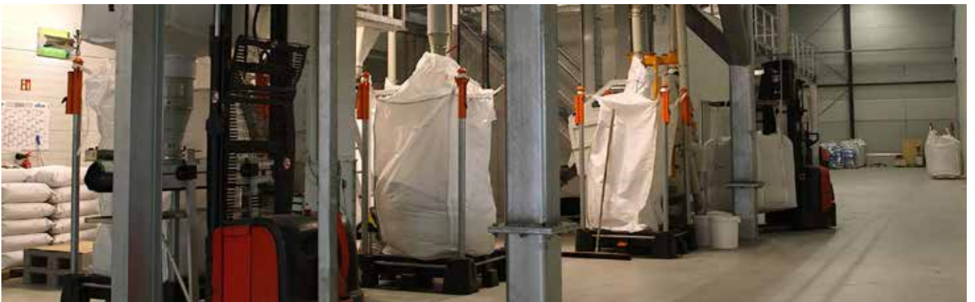
Ground floor view of the Hemp Factory production line. The facility is the biggest hemp food processor in Central Europe.
