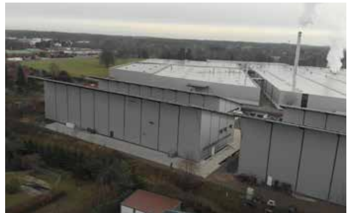
Hemp Factory is located at Borken, Germany near the Dutch border
