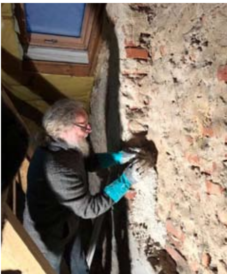
Belgian natural builder Wolf Jordan demonstrated wall construction and the application of hemp-lime as finishing material at Deep Green Building I 2018.
