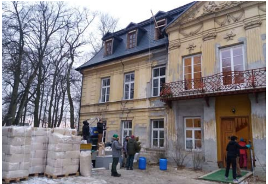
Hempcrete was mixed outside with warm water, and hoisted to the attic by block-and-tackle.
