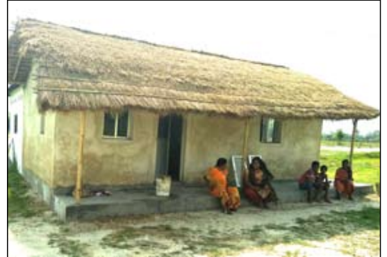
A SHIV-built family dwelling from hempcrete; on a mango tree farm.
