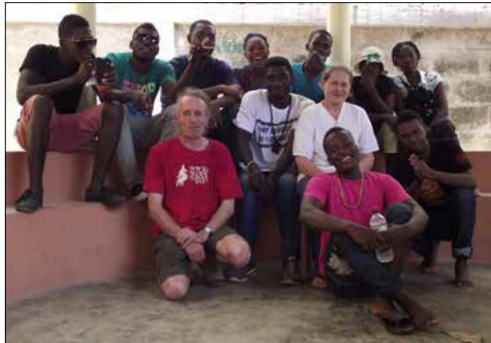
Steve Allin and Finnish architect Ritva Laurila with an extended work crew at the Port au Prince site. (Right) Workers apply hurd as fill-in roof insulation.
